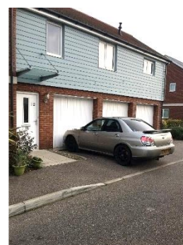
An example of poor design, resulting in footway obstruction due to an overhanging parked vehicle.
